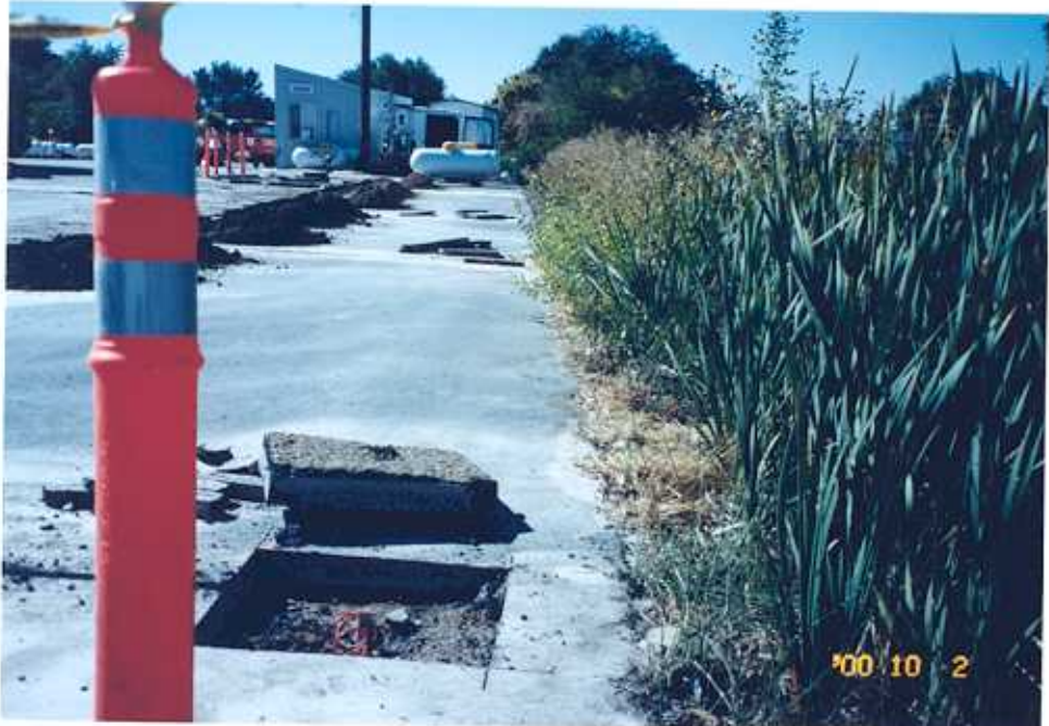
Below: Drilling and installation of components complete, SME components are ready for connection and the surface seal.
