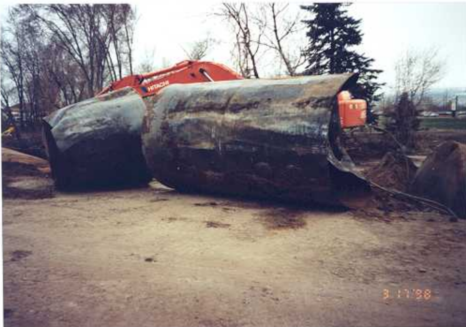
Below: Failed underground storage tank broke in half during removal.
